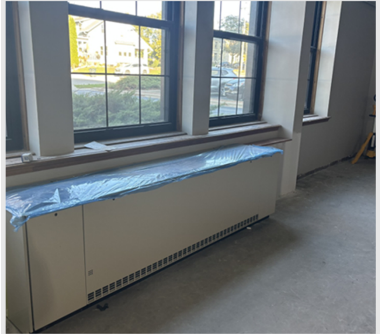
Unit ventilators have been installed in 1 st and 2 nd floor classrooms.
